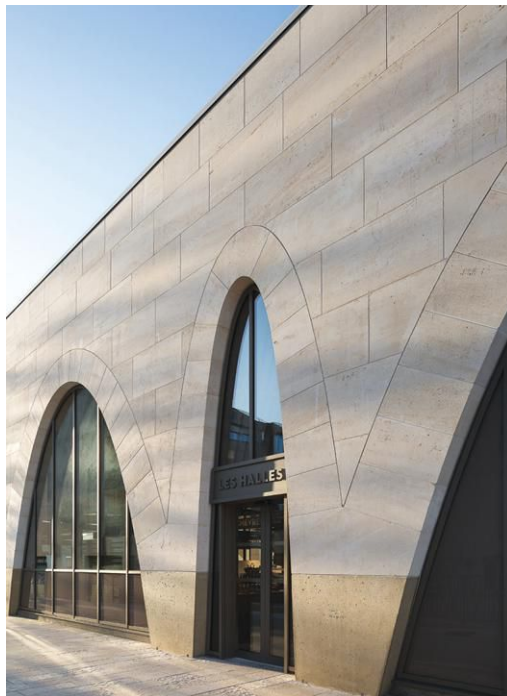
The market hall uses locally sourced stone and timber (above and above, right). The arches are set in place with support frames (right and far right).
