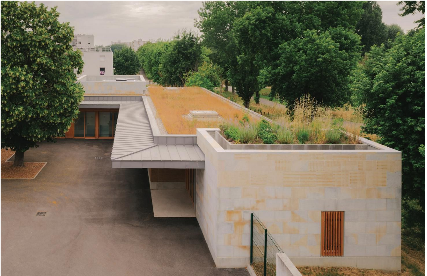
The use of multicolored stone kept costs down (above). The roof is built of cross-laminated timber (left).
