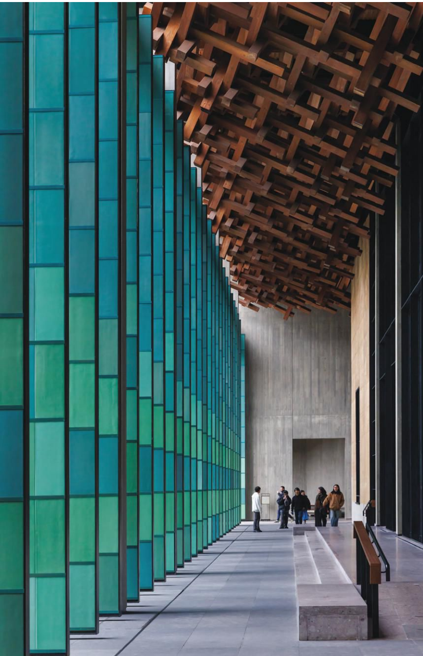
Celadon-clad screen walls line the campus's arcades, and they can be rotated and moved.
