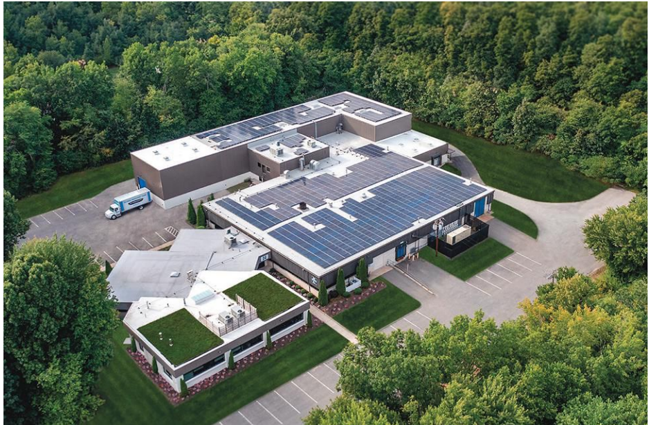
The addition and renovation includes a living roof and photovoltaics.
